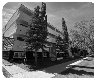
Mainstreet purchases buildings along bike paths and retrofit the properties with bike racks and scooter parking pads to empower our tenants to live sustainably without sacrificing convenience, and demonstrate that we understand what they're looking for.
