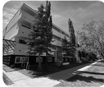
Mainstreet purchases buildings along bike paths and retrofit the properties with bike racks and scooter parking pads to empower our tenants to live sustainably without sacrificing convenience, and demonstrate that we understand what they're looking for.
