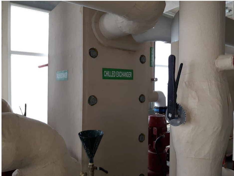
Photo 26 Heat exchanger
