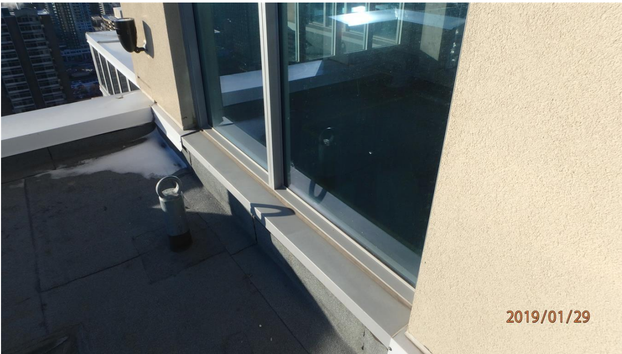
Photo 16 Typical metal flashing
