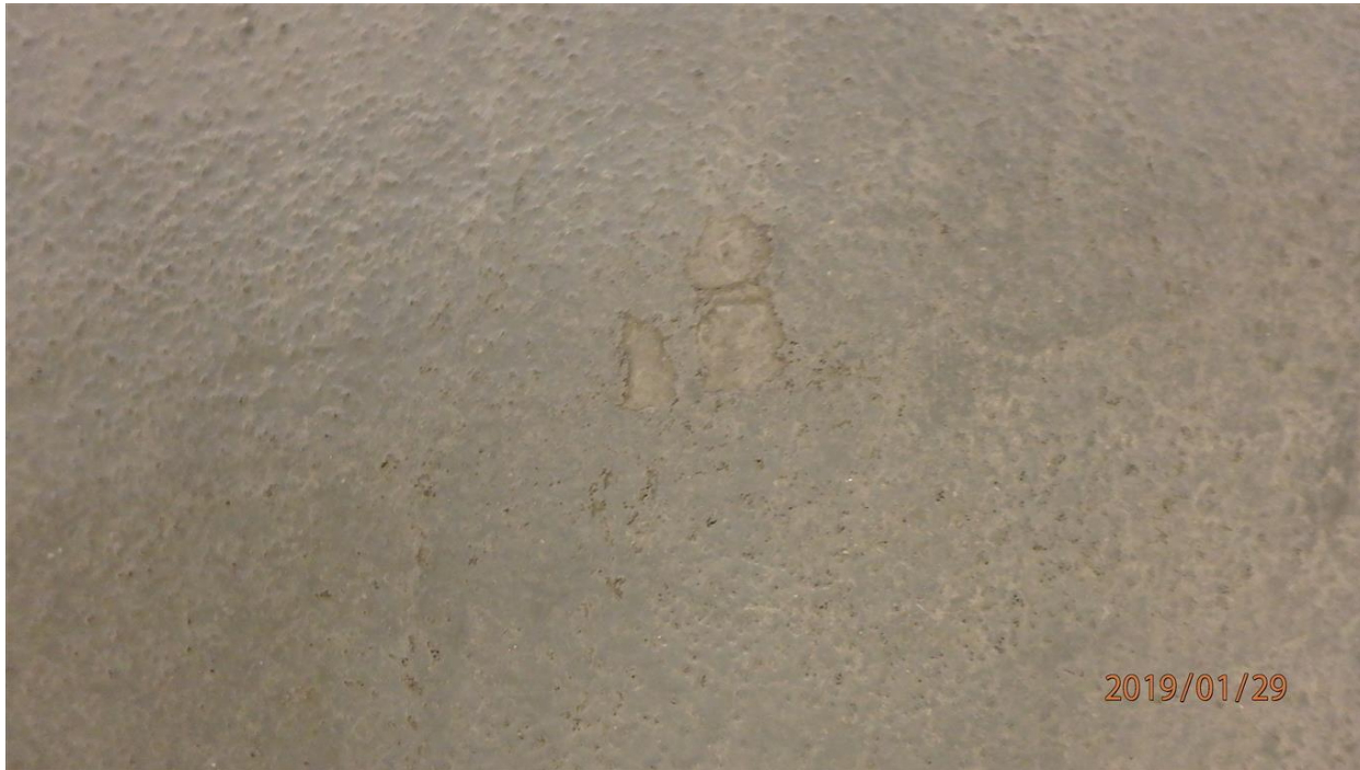
Photo 9 Damage to parkade membrane
