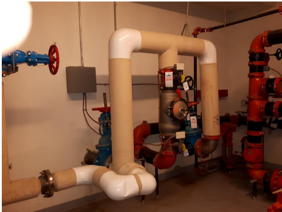
Photo 4 Water entry room
