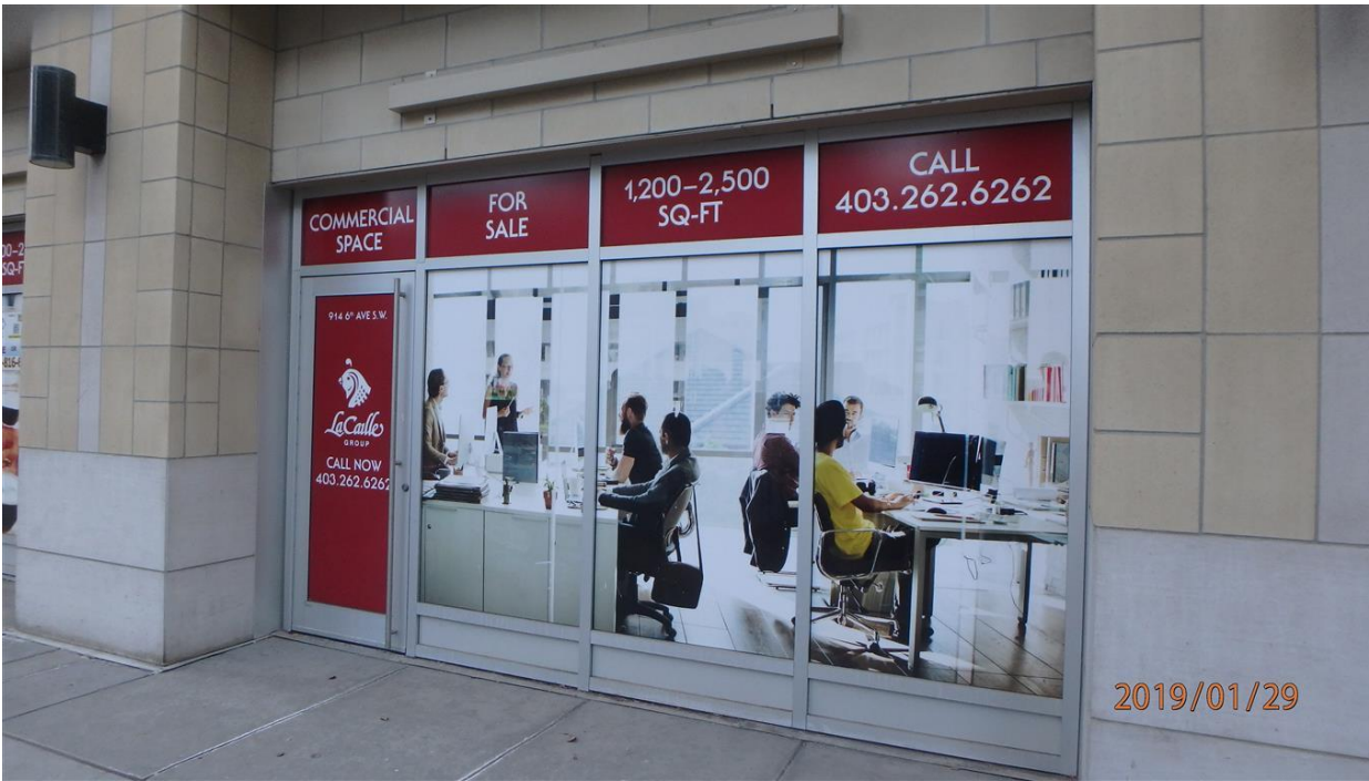
Photo 11 Exterior curtain wall
