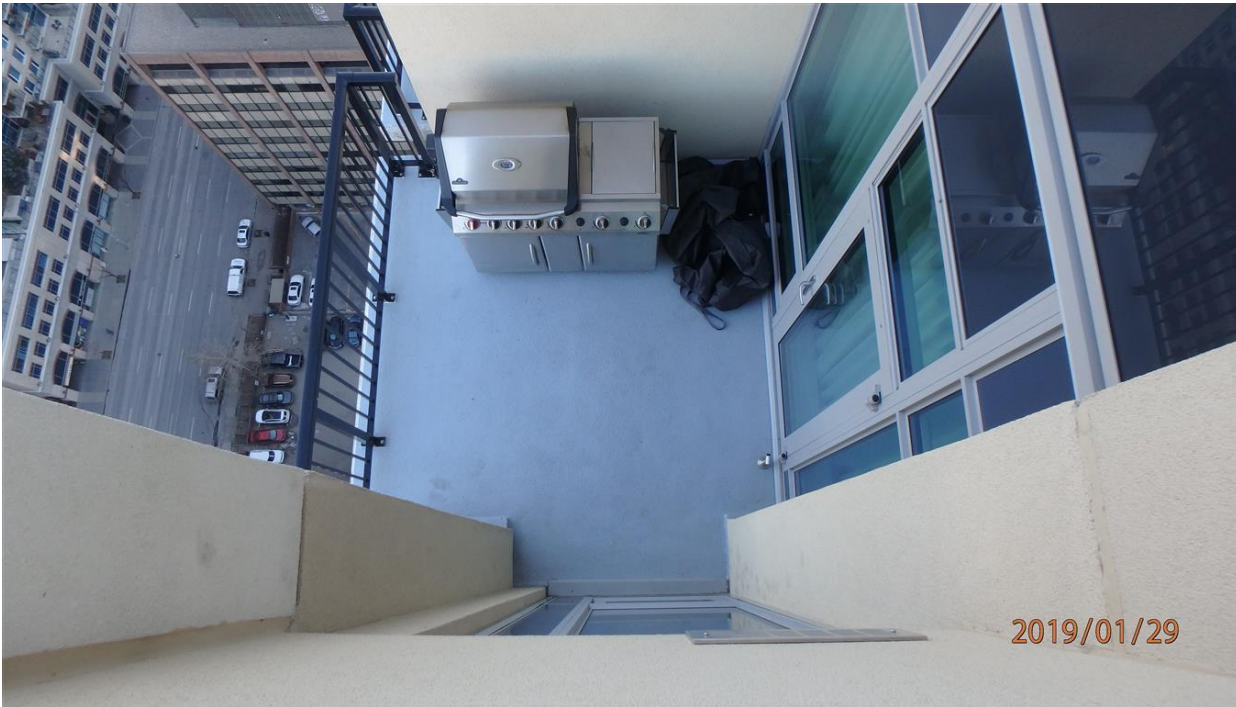
Photo 1 Typical balcony and aluminum railings
