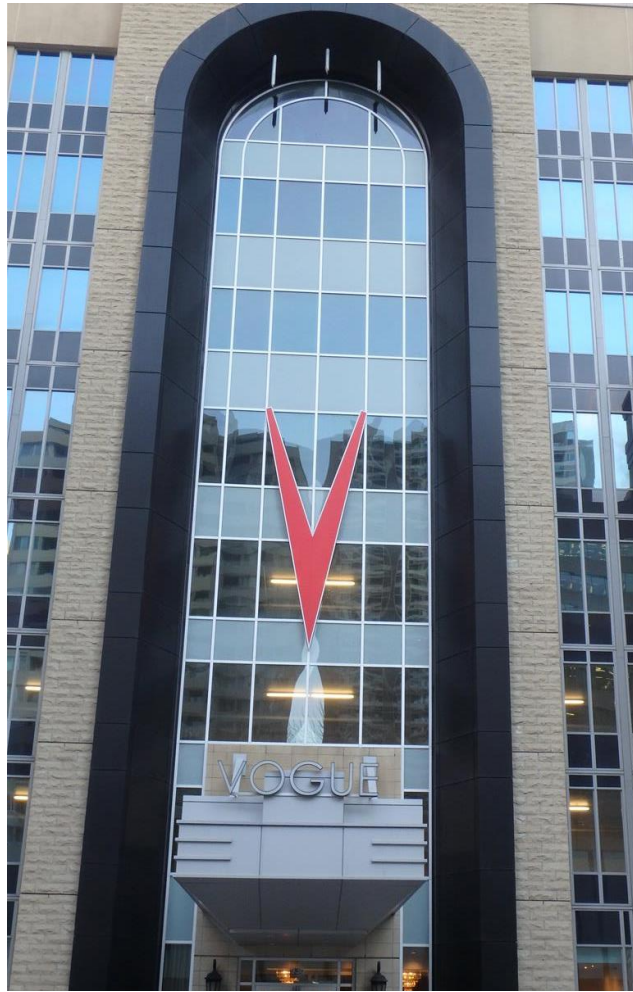
Photo 5 Composite metal panels at front entrance
