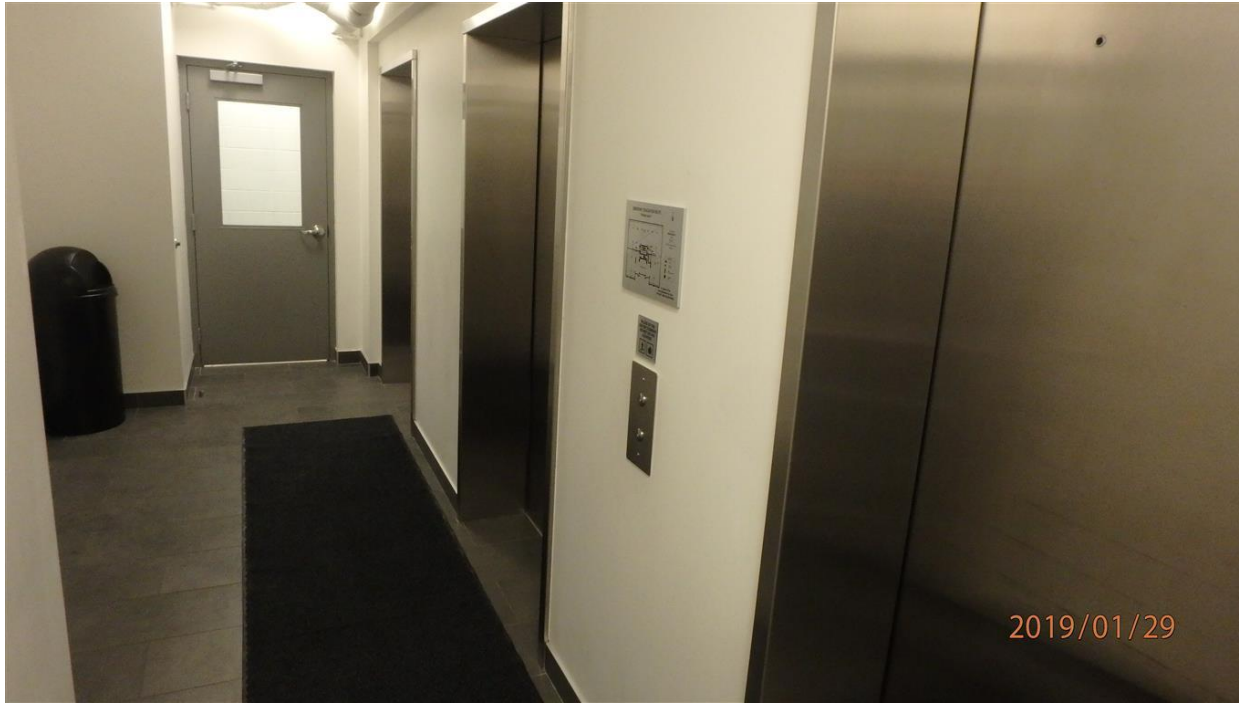
Photo 21 Typical parkade elevator lobby
